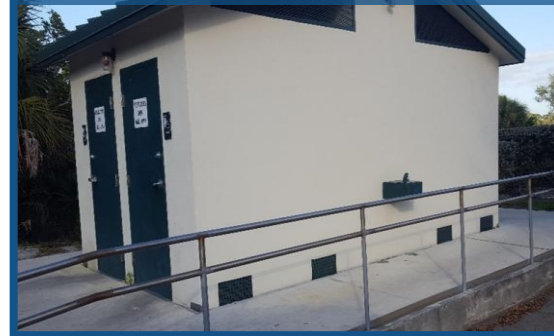
Flood Vents on a Park Restroom
