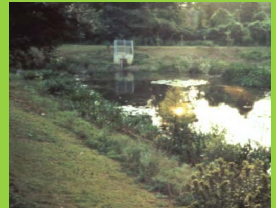
Wet detention pond
