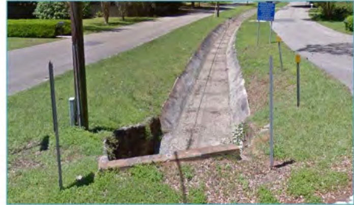
3. GWD – San Luis Road – Concrete Ditch
