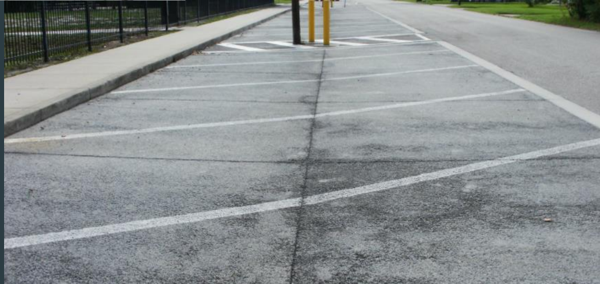
Pervious concrete along W Estrella St
