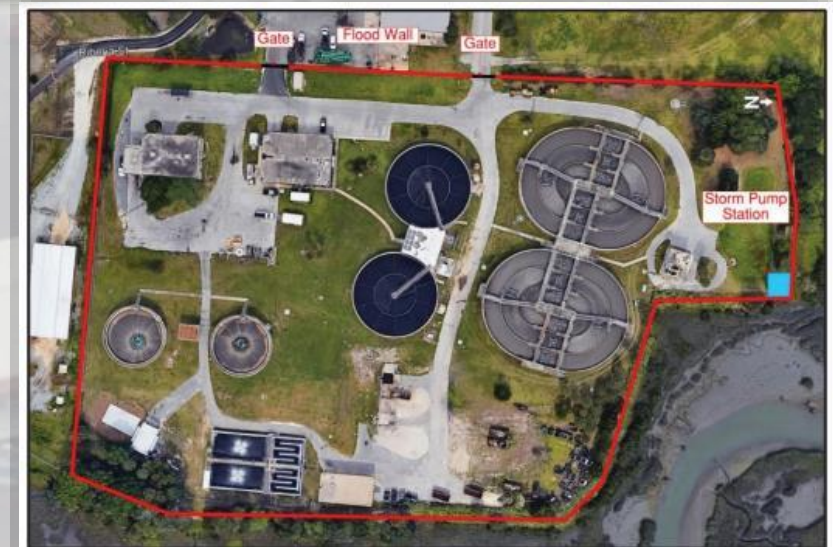
Figure 10: Perimeter Flood Wall and Pump Station
