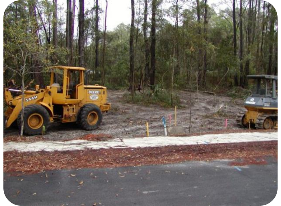
Limited Site Clearing
