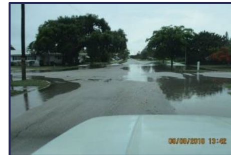
Lack of Drainage 2 nd Street Corridor)
