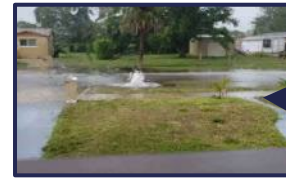
Ilex Court Inlet Surcharge
