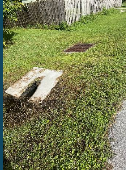
Culverts and inlets
