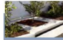
FILTRATION TREE BOX
