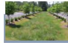
FILTRATION BIO-RETENTION SWALES
