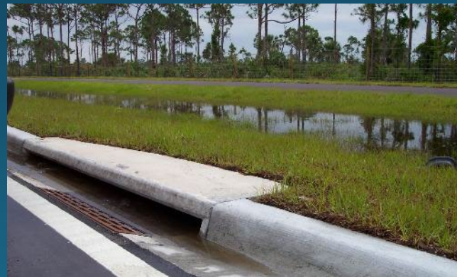
Curb and Inlets
