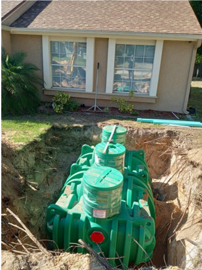
Septic Tank Upgrade
