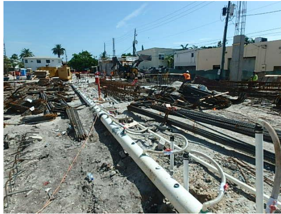
Well-point dewatering system
