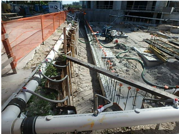
Well-point dewatering system
