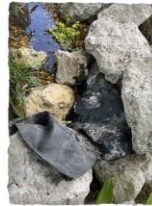
Build bottom shore up wall for support of basin
