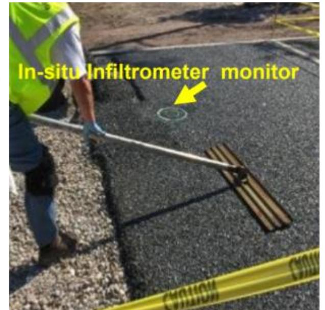
In-situ Infiltrometer monitor
