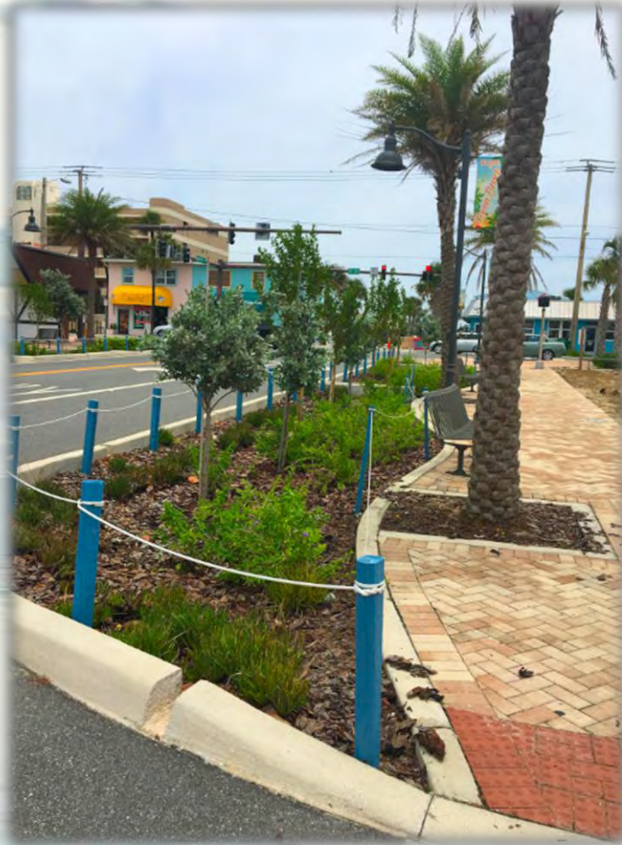
rain garden foot traffic & curb flow bypass
