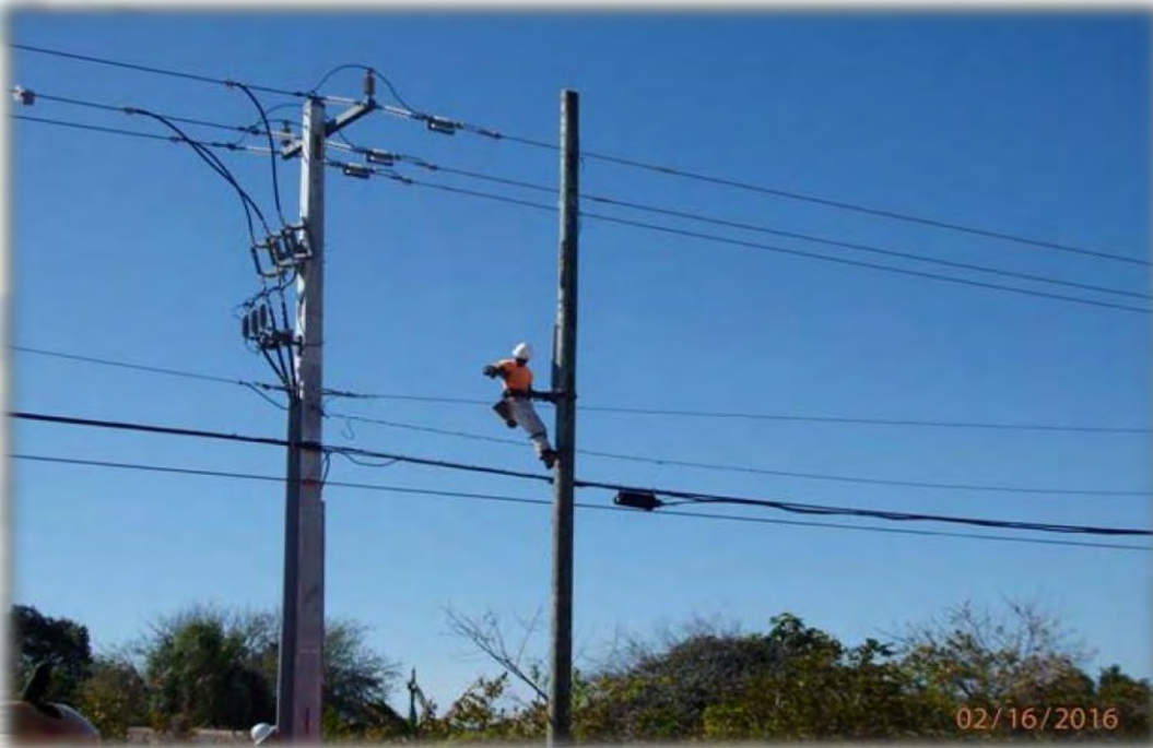
upgraded FPL power lines
