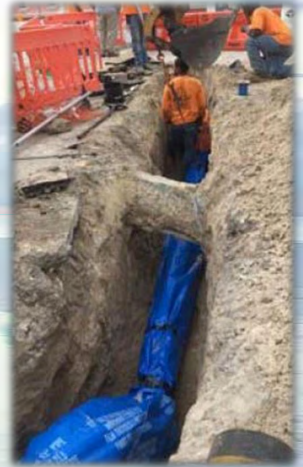
upgraded water lines
