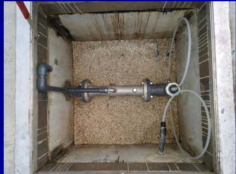
Venturi for Alum Addition
