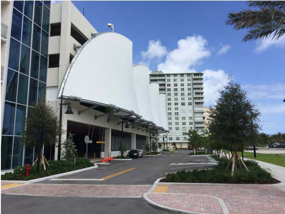
Pompano Beach Parking Facility
