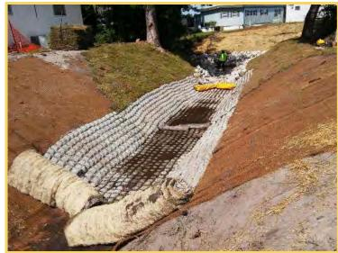
Articulated concrete block and Flexamat™ for slope stabilization
