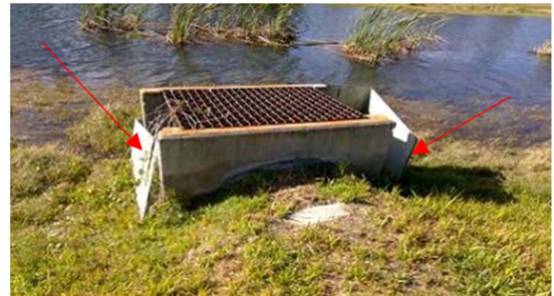
Skimmer is broken – poor condition
