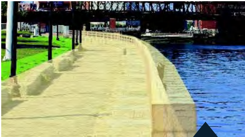
HARBORWALK FLOOD BARRIER
