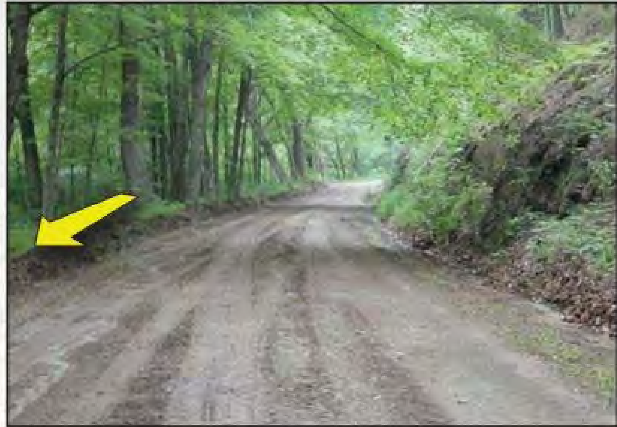
Figure 4.15—The berm was created by recent grading. Removing the berm and crowning the road allows sheet flow into the vegetation to the left.
