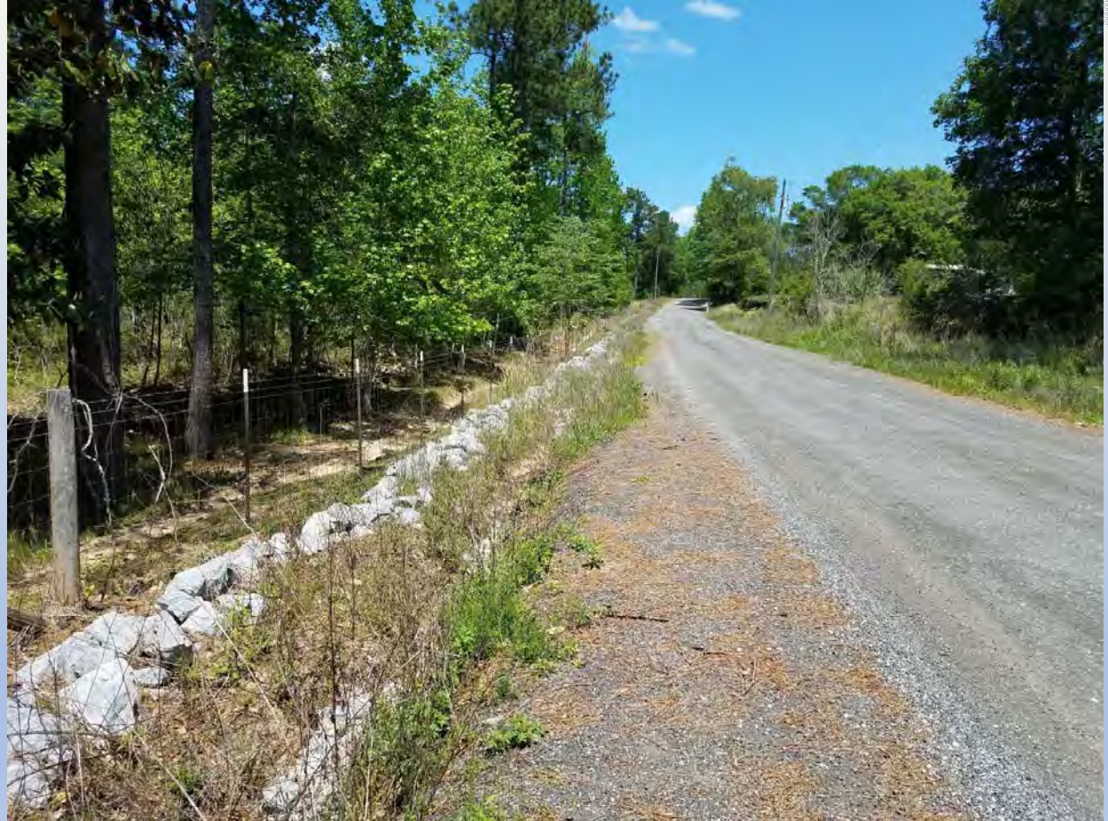
Roadway aggregate and riprap ditch in Walton County, FL
