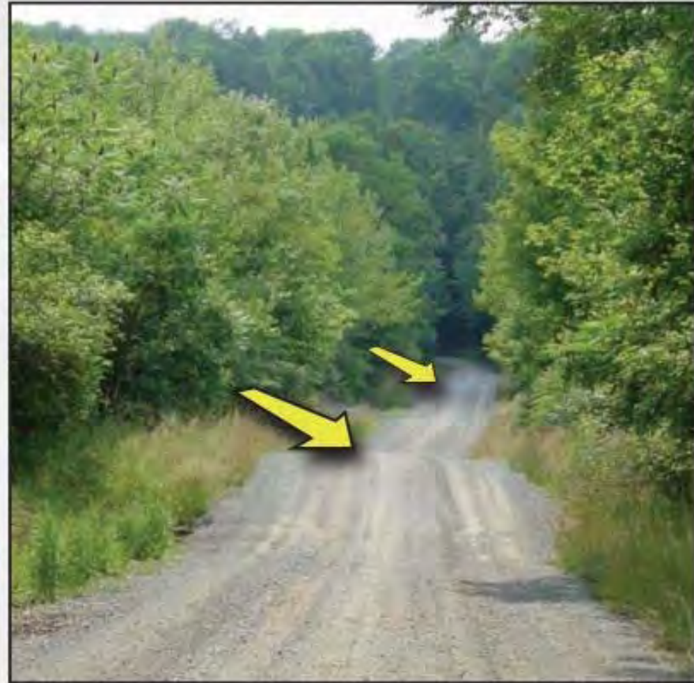
Figure 3.7—The two grade breaks pictured here prevent water from flowing down the road, even if the road's crown were to be lost.
