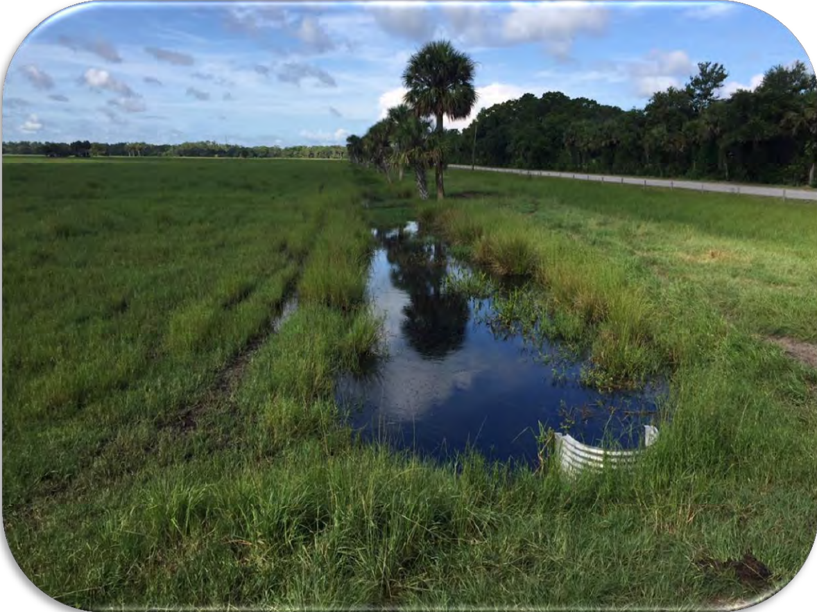
Perimeter ditching to retain water on-site
