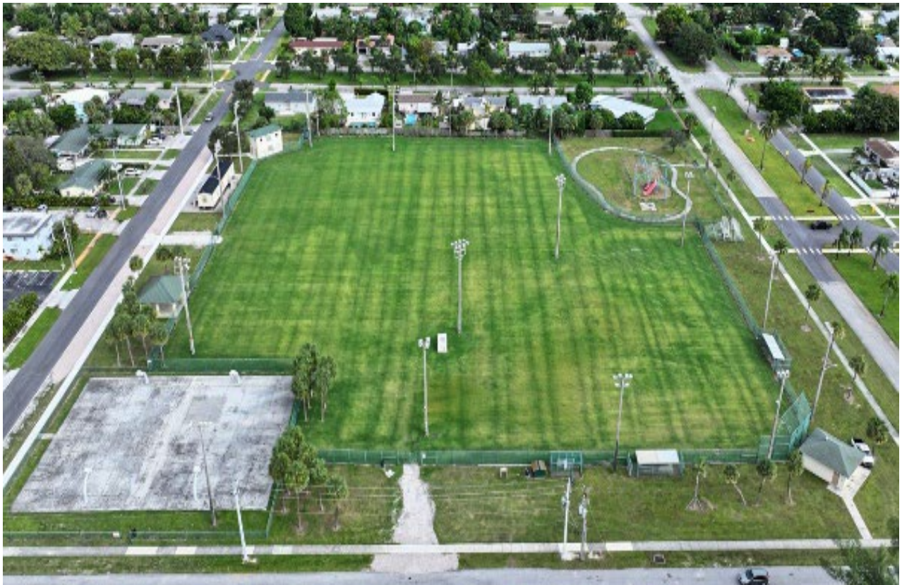
Fully restored athletic field following completion of underground construction, demonstrating successful integration of large-scale green stormwater infrastructure within an active community park.
