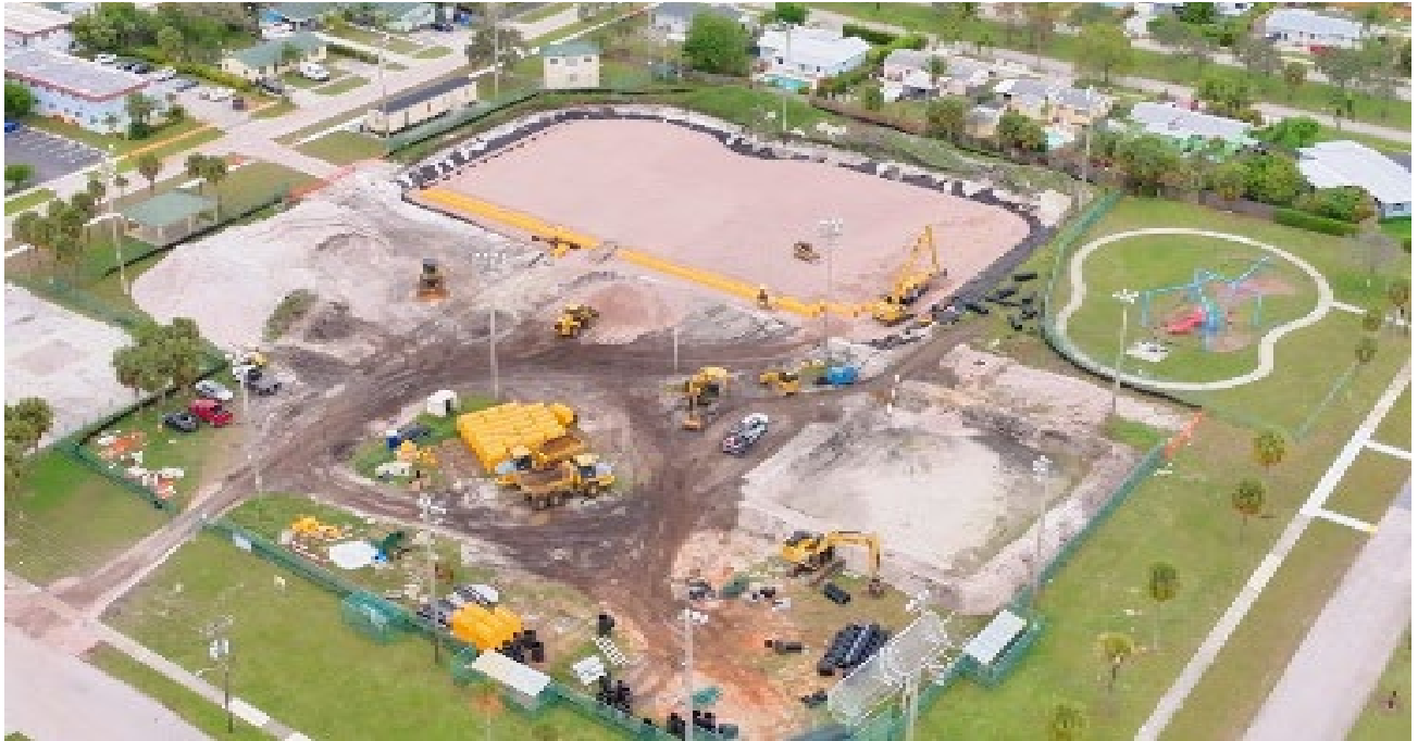
Installation of underground detention and filtration chambers beneath the athletic field, demonstrating the scale of the infrastructure while maintaining careful phasing to minimize disruption to surrounding neighborhoods.
