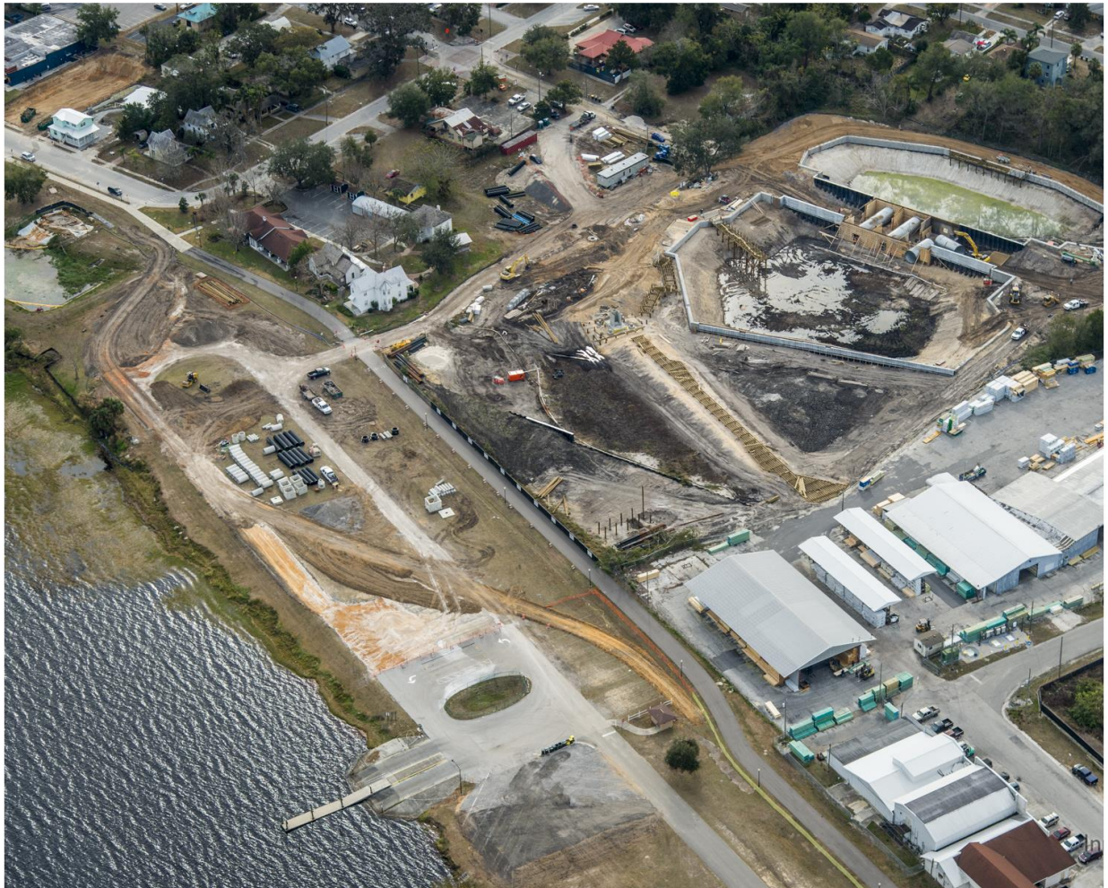
Construction of the Site
