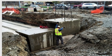
StormTrap Stormwater Management Treatment System - US Bank Stadium West Plaza - Minneapolis, MN Robert Daw
